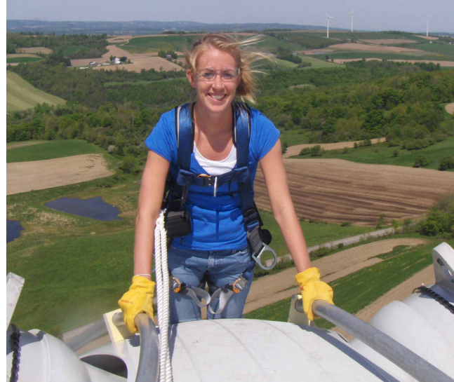
GE Wind Energy Learning Center employee, 250 feet in the air servicing a GE 1.5 MW Wind Turbine.
